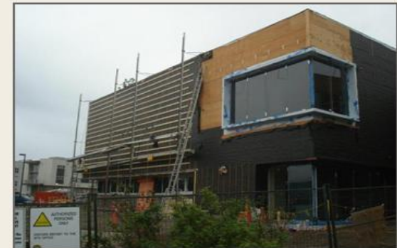
Lecture Theatre - 30 days from completion
